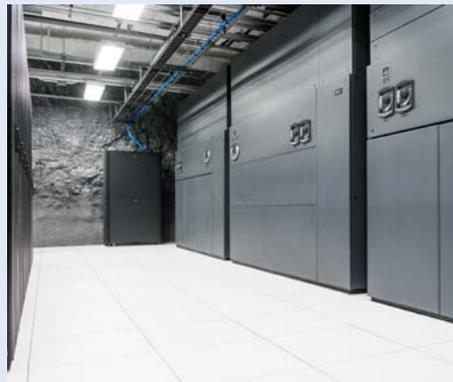
STC provides efficient power distribution to the floor with 225 W/SF and features N+1 redundant power systems with concurrent maintainability.
